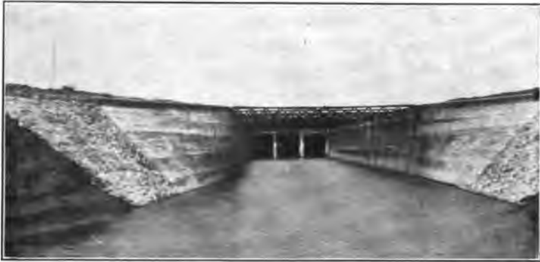
FIG. 152.—Inlet to Rawhide Siphon, Interstate Canal, Nebraska-Wyoming.
